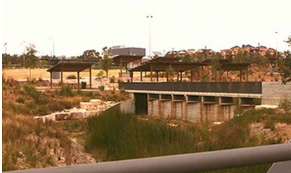
Photo: Blacktown Showground Precinct
