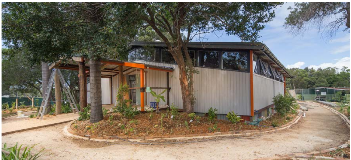
Image: Warringah creative space near completion
