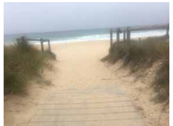
Fabricated pathway linking to existing concrete path
